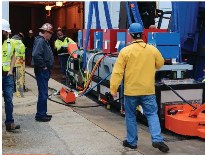
Argonne National Laboratory used an air bearing system with power drives to move long and heavy equipment into the facility.
