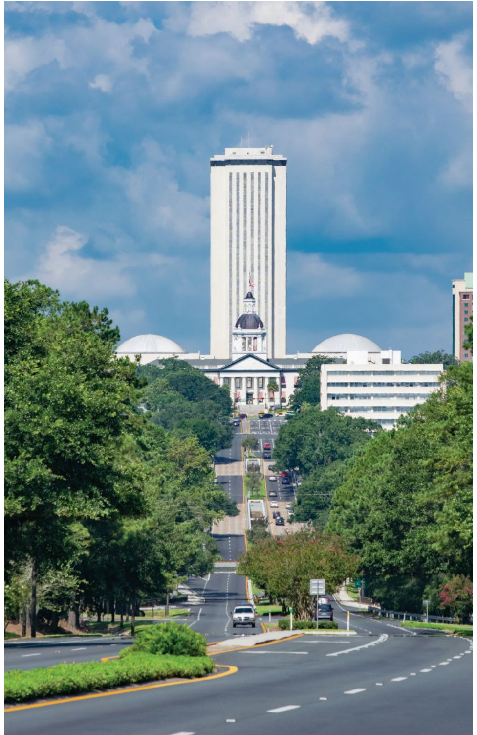
The Florida State Capitol building and Apalachee Parkway.
