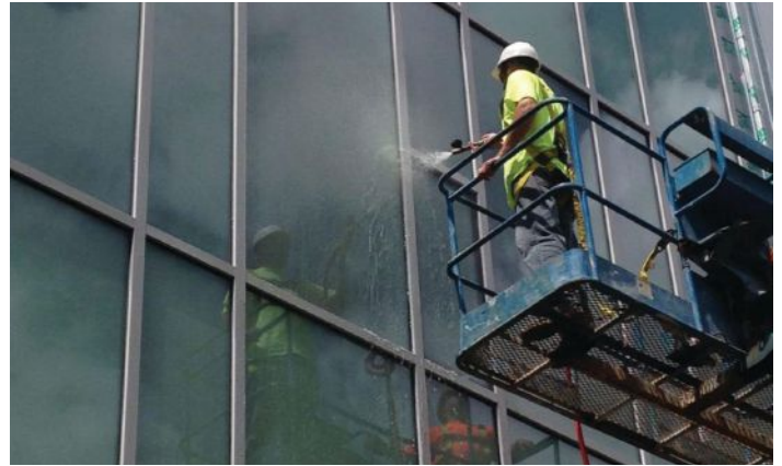
Hose spray testing can be used to identify water infiltration sources.
