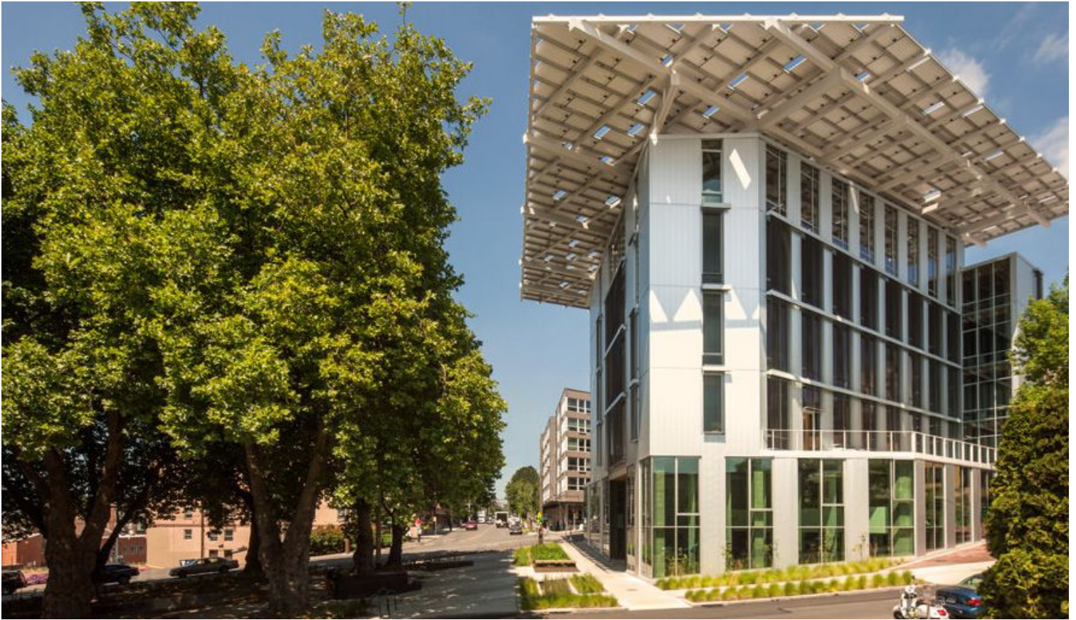
Bullitt Center, Seattle, Washington, USA
