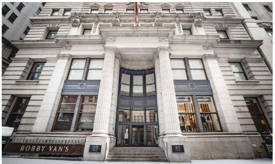
Window inserts are barely visible from the inside of landmark New York City building, blocking drafts and city noise.
