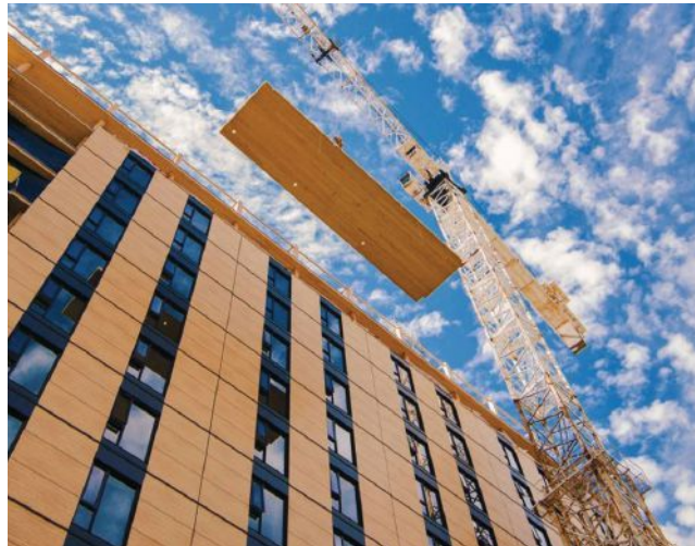
UBC Brock Commons- 18 Story Tallwood House, Vancouver, BC, Canada; Structurelam Mass Timber Corporation
