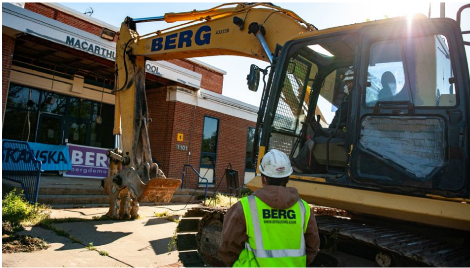
ACPS is building a new facility for Douglas MacArthur Elementary School
