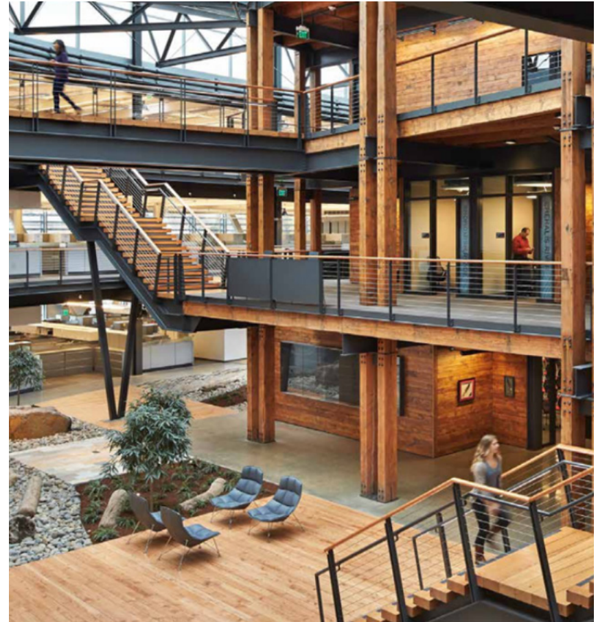
Source: U.S. Army Corps of Engineers Headquarters building utilizing 300,000 board feet of structural and non-structural lumber from an adjacent warehouse deconstruction. | https://www.gsa.gov/cdnstatic/GSA_FCS_Press_Book_email.pdf
