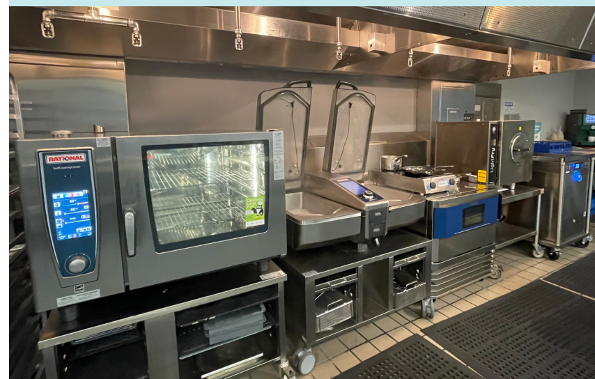
FIGURE 5.19: A HIGH TECH ALL-ELECTRIC KITCHEN LINEUP WITH COMBI OVEN, INDUCTION COOKTOP, FLEXIBLE BRAISING PAN, BLAST CHILLER, HOT AIR FRYER, AND HEAT RECOVERY DISHWASHER
