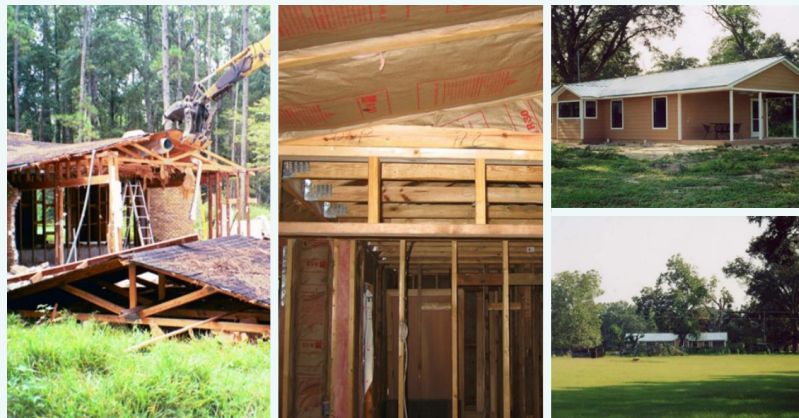
Images of an undamaged 1970s Florida floodplain buyout home being deconstructed. The lumber was used, under existing building codes, to rebuild HUD Section 8 Affordable Housing inland. Photos: Brad Guy
